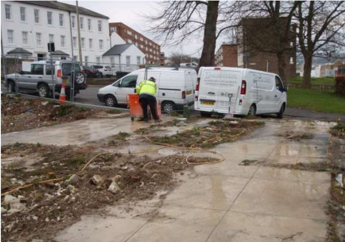
Plate 14. Diamond sawing concrete slab (looking north-west)
