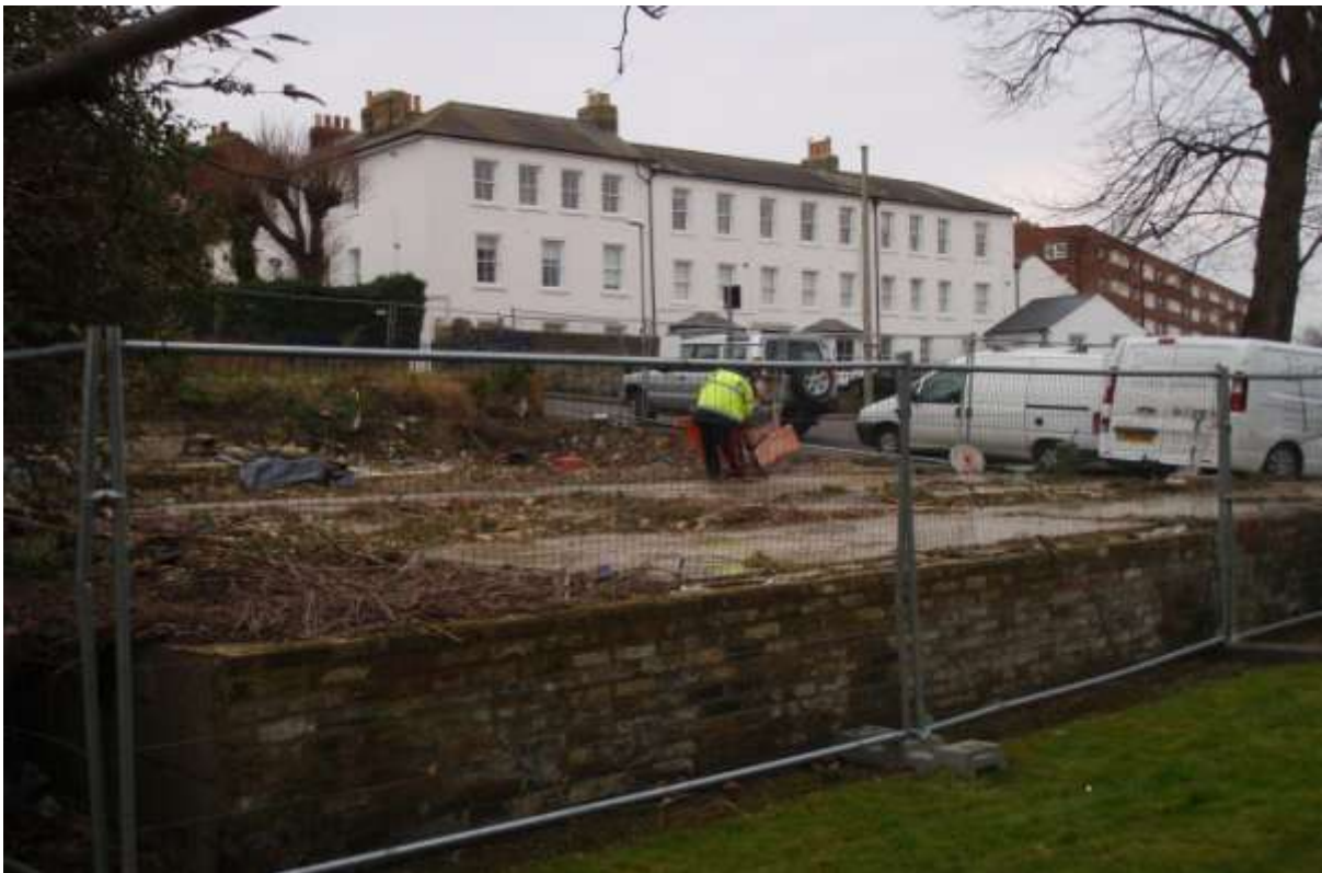
Plate 15. Diamond sawing concrete slab (looking west)
