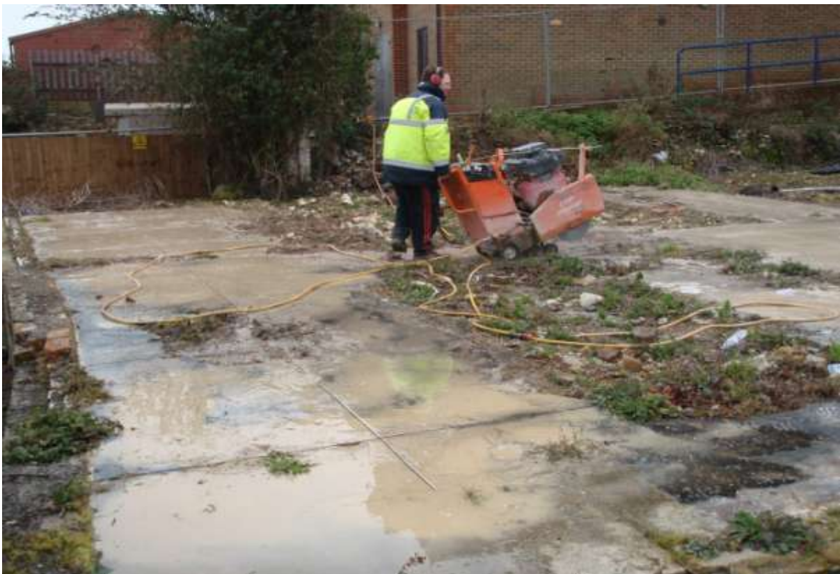
Plate 13. Diamond sawing concrete slab (looking south)
